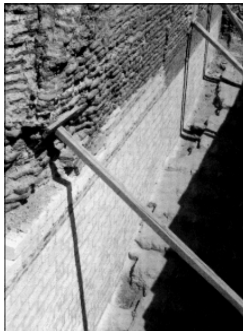
Fig. 3. Cisterns. Western wall of the corridor after restoration (Photo W. Kołtąj)
