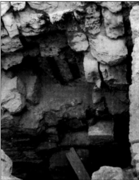
Fig. 4. Cisterns. South double wall before restoration (Photo W. Kołtątaj)
