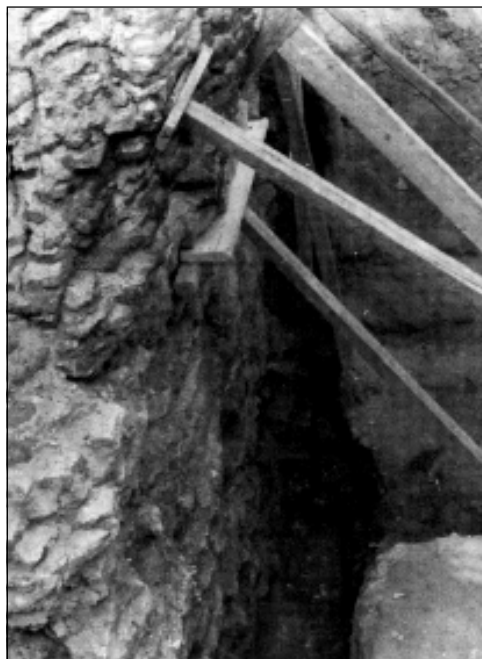
Fig. 2. Cisterns. Western wall of the corridor before restoration (Photo W. Kołtąj)
