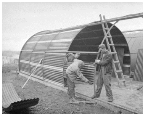
Rys. 2.1. Hale systemu Quonset Hut (1942) [3]
